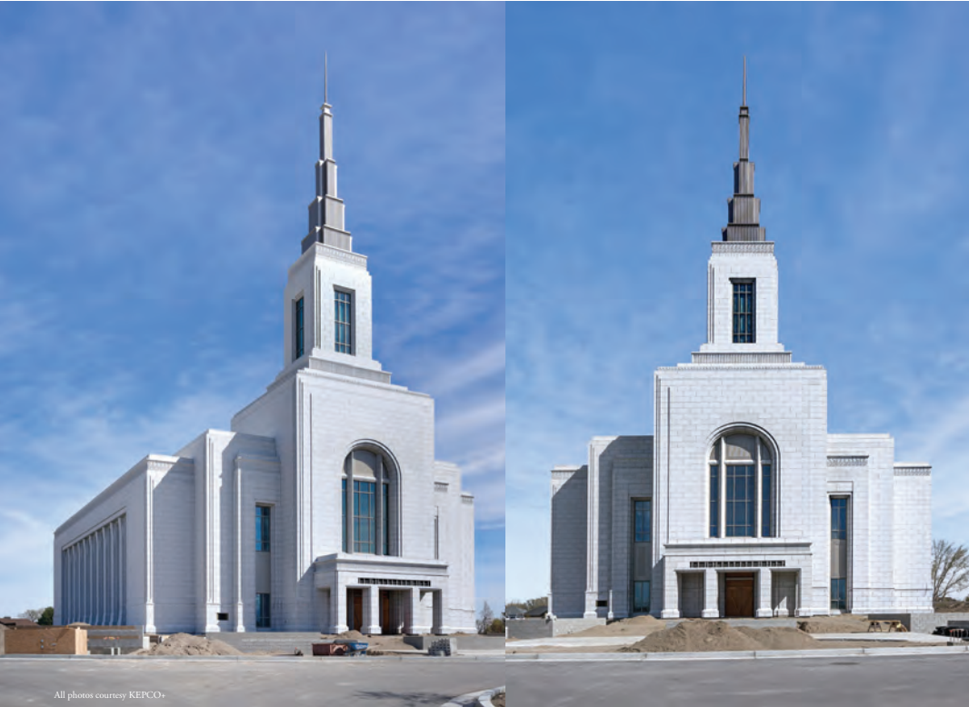
All photos courtesy KEPCO+
