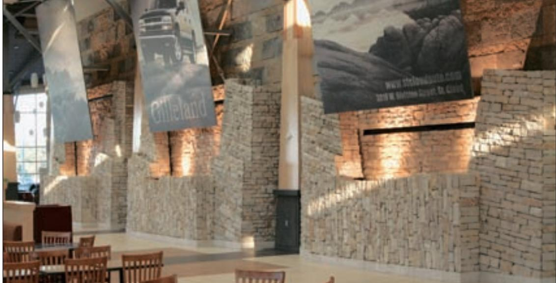
is affixed to the wall by applying mortar to the back of the stone and pressing it to the wall. On dry interior applications, thin stone can also be adhered to the back-up wall using special epoxy adhesives approved for thin stone applications.
