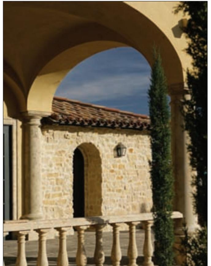
ABOVE BOTTOM: In the Southwest, the very same Natural Stone Veneers International Sydney limestone thin stone used on the Traverse City Condo is given a completely different look when set with an appealing overgrout. The overgrout yields a rustic, old world feel to the veneer.
