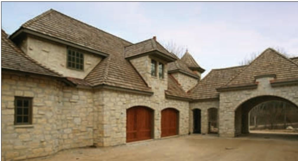
LEFT: In areas of the exterior that couldn't support a full thickness stone load without additional support, the walls were plastered and thin stone was blended into the mix.
