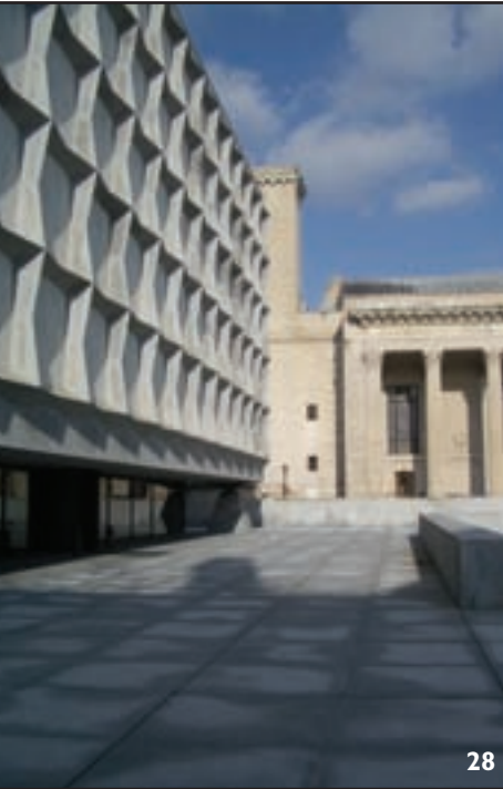
Photo courtesy of E.F. Prokop
