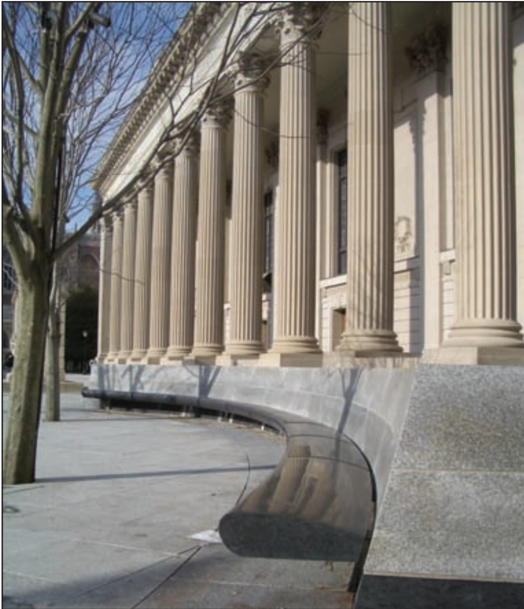
ABOVE: Benches were constructed of four vertical segments of split-face stone: an initial stratum of Woodbury Granite is followed by a strip of Black Peribonka which forms the seat; a second strip of Woodbury is topped with a Woodbury cap.
