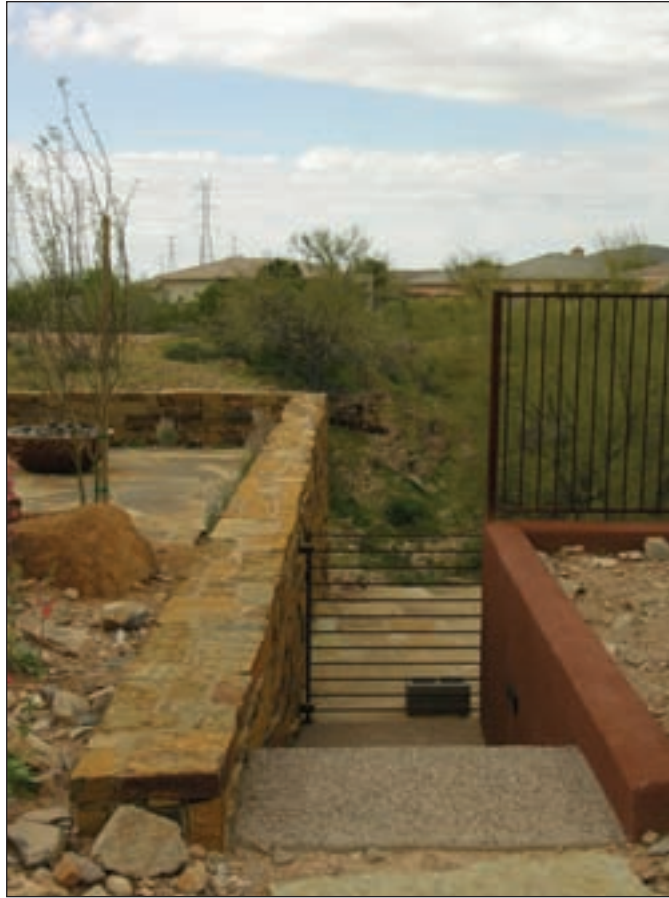
LEFT: This dry stack stone wall reaches out toward the existing desert wash. Exposed aggregate steps form the access from the wash to the upper lawn. Photo courtesy of Sunni Jackson and Urban Earth Design LLC
